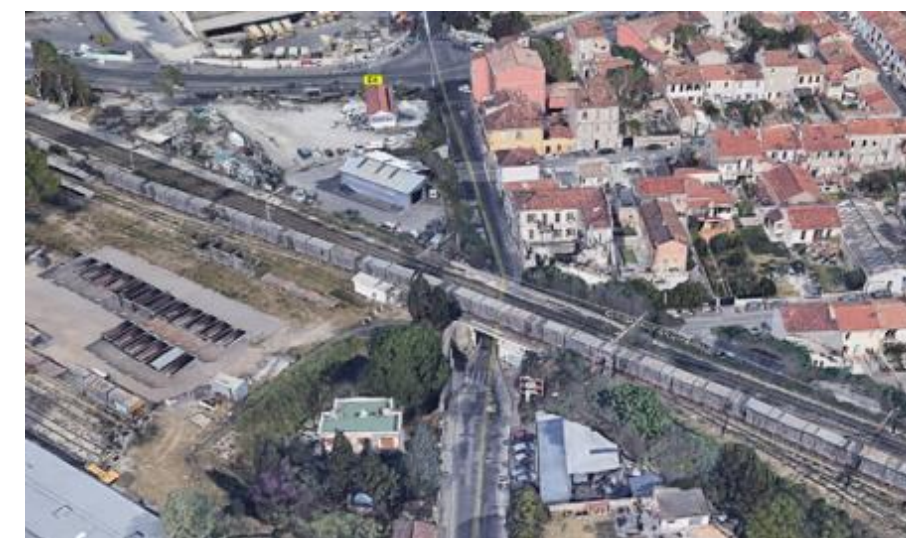
Figure 43 : Pont rail de l'avenue Ibrahim Ali (Google Earth, 2021)
